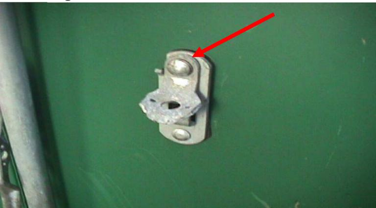
Seals should be affixed to the right door on the hasp that has the welded rivet.
